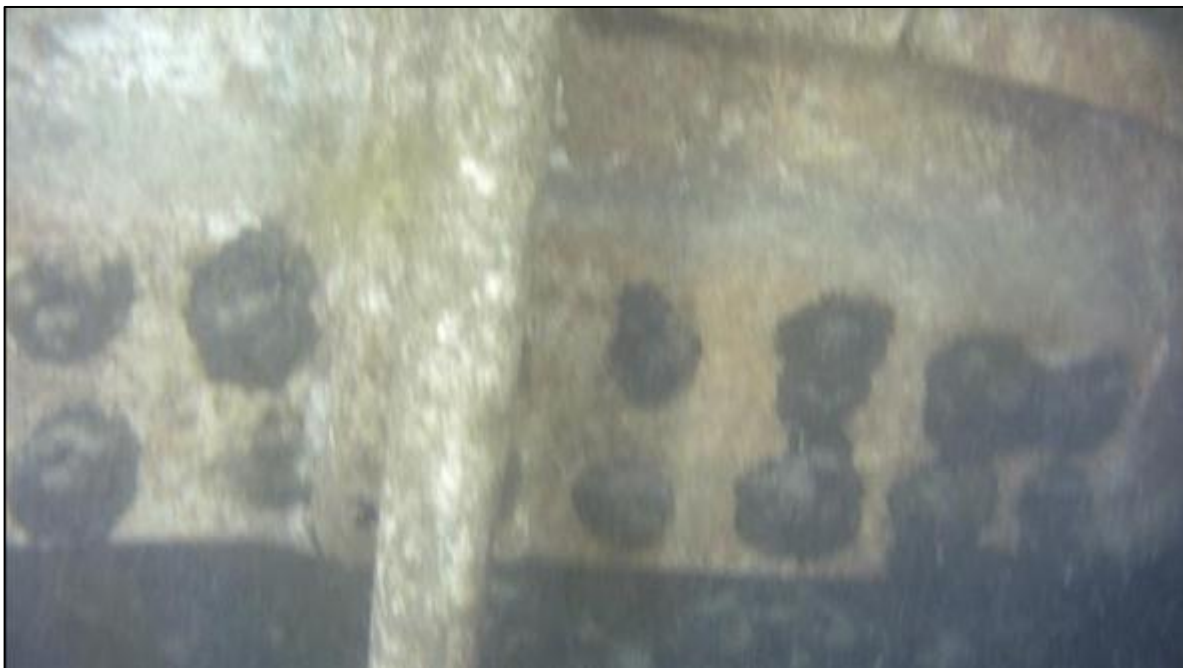
Figure 32 - This Image shows the Twin Lines of Rivets that join the Two Parts of the Conning Tower
