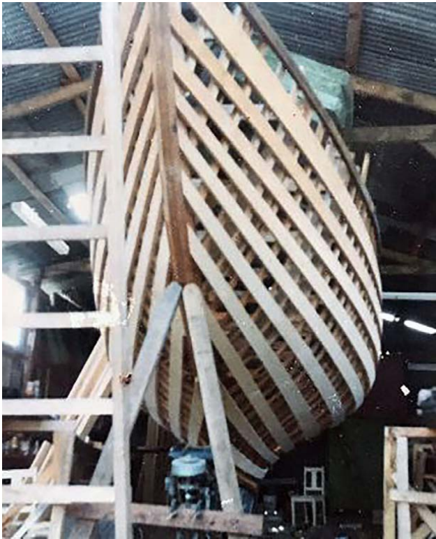
Sagan under construction (Photo courtesy Derek Shields)
