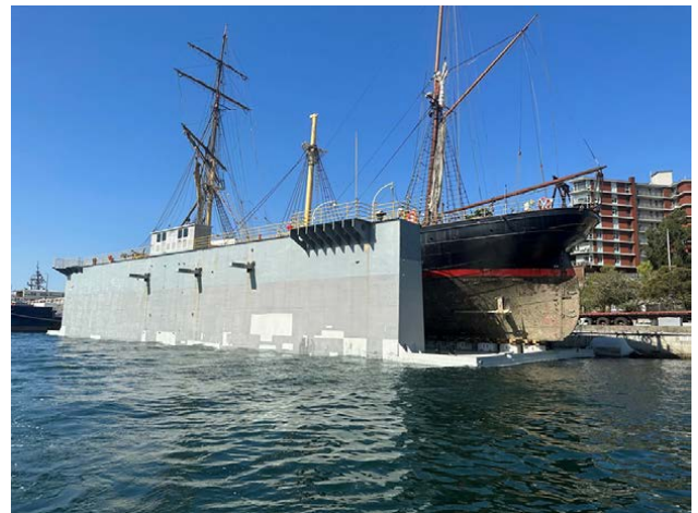
Aft overhang for removal of rudder (Photo courtesy Sean Langman)
