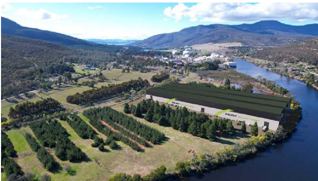
The site of Incat Tasmania's new shipbuilding facility in the Derwent Valley, Tasmania (Illustration courtesy Incat Tasmania)
