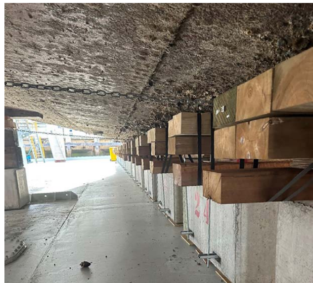
Line of keel blocks (Photo courtesy Sean Langman)
