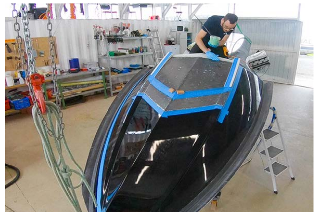
Adding an extension to the (upside-down) centre hull (Photo from SP80 website)
