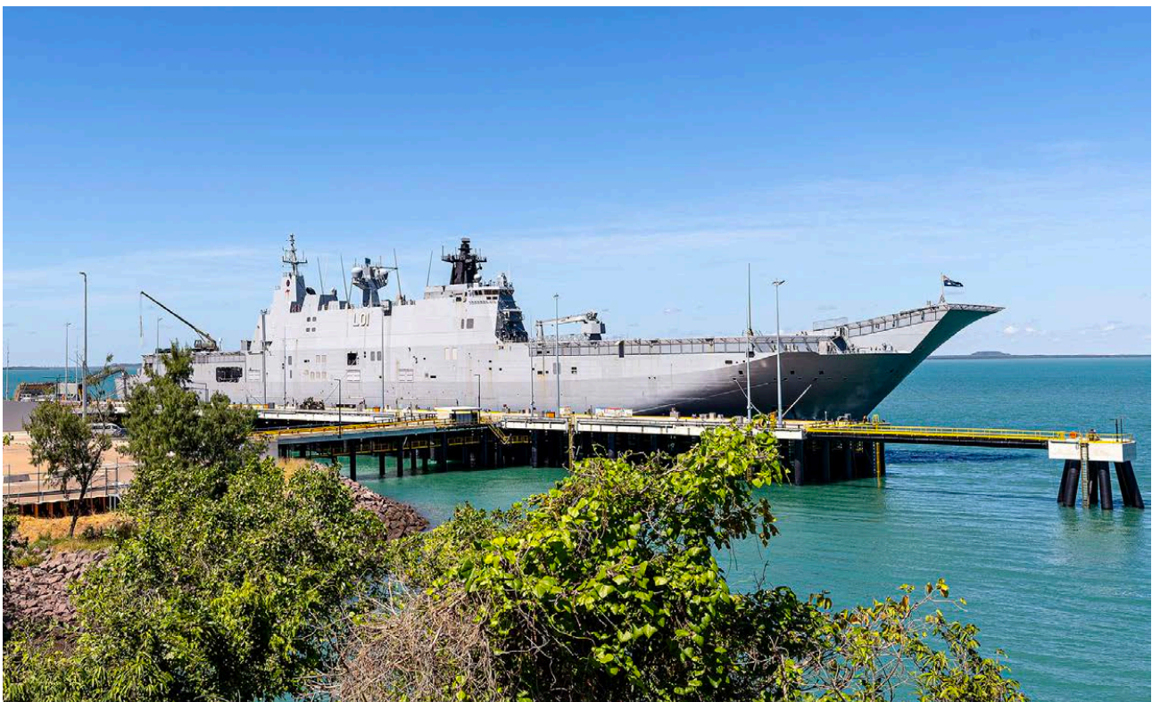
HMAS Adelaide recently conducted the first Landing Helicopter Dock-sized berthing alongside the brand-new Kuru Wharf at HMAS Coonawarra , Darwin. This event marks a significant achievement in the ongoing upgrades of waterfront facilities at the Larrakeyah Defence Precinct. The Kuru Wharf measures approximately 250 m in length, with two approach jetties. The new wharf is now able to support up to LHD-size naval vessels, providing game-changing capability support in the north (RAN photograph)
