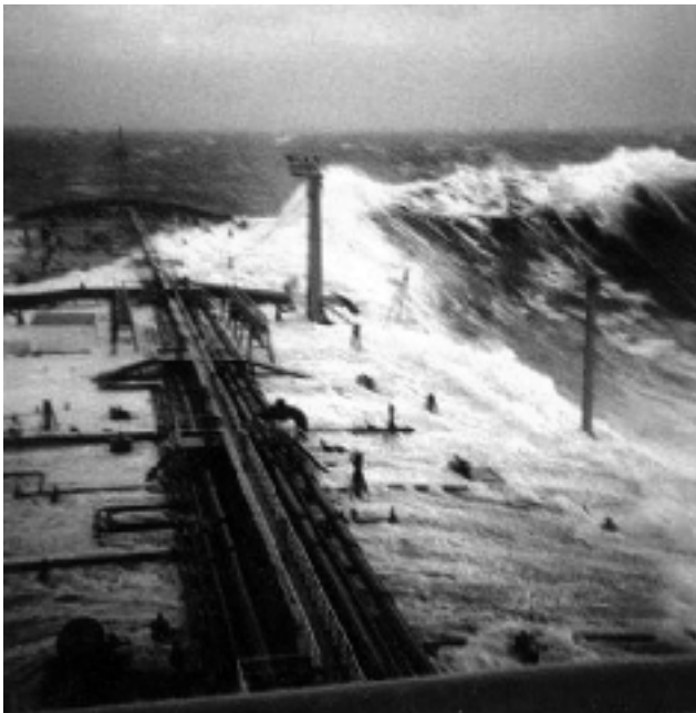
This rare photo of a rogue wave was taken by first mate Philippe Lijour aboard the supertanker Esso Languedoc during a storm off Durban in South Africa in 1980. The mast seen to starboard in the photo stands 25 m above mean sea level. The wave approached the ship from behind before breaking over the deck, but in this case caused only minor damage. The mean wave height at the time was between 5 and 10 m. (Photo Philippe Lijour)
