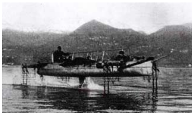
Figure 6 — Photograph of hydrofoil driven by water propeller running foilborne
