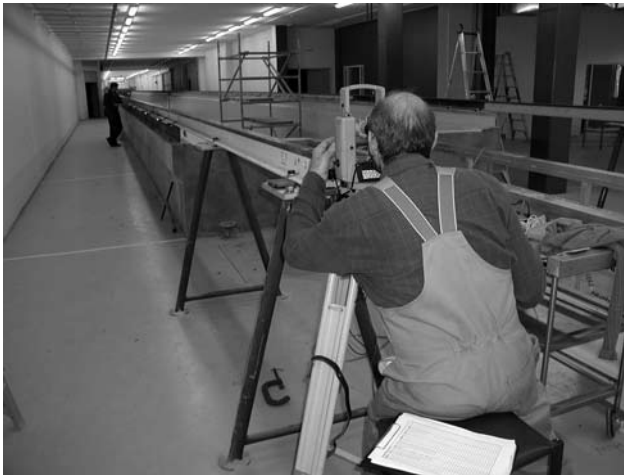
Aligning the carriage rails (Photo courtesy AMC)
