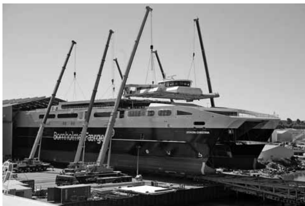
Erecting the superstructure of Leonora Christina (Photo courtesy Austal)
