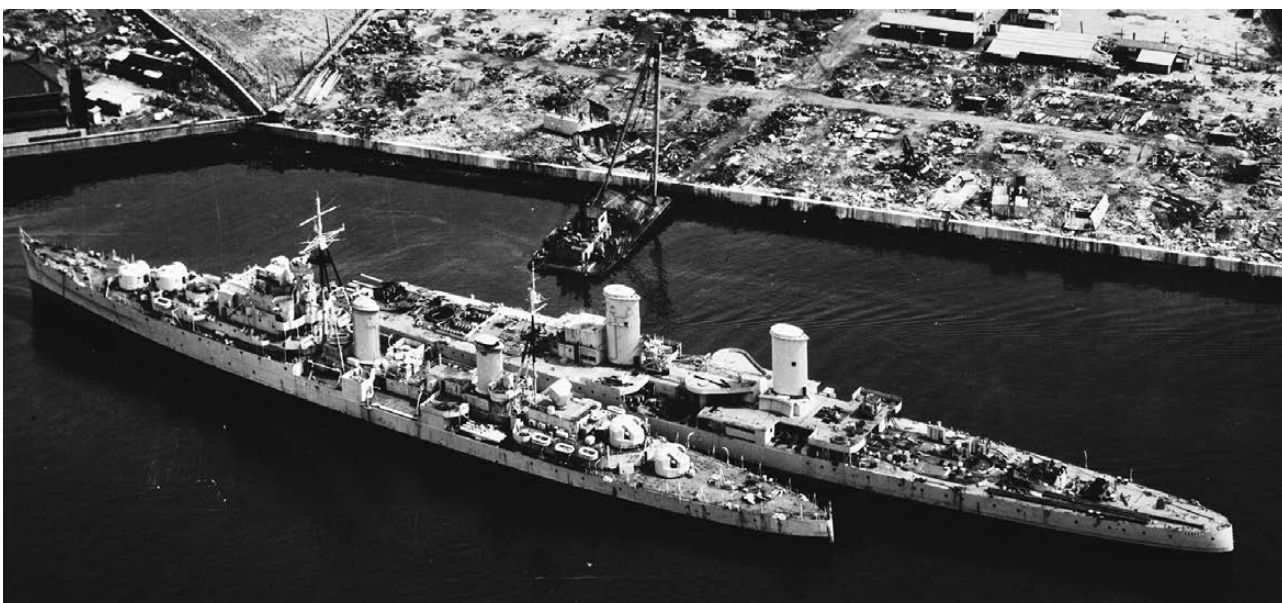
Demolition of Hobart well underway at the shipbreakers in Osaka. The cruiser alongside on her port side is the Dido-class cruiser ex-HMNZS Black Prince (RAN Historical Collection)
