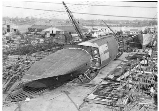
A PC hull being rolled over at Defoe during WWII (Photo courtesy Bay County Historical Society)
