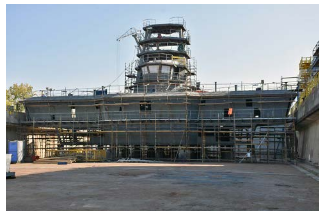
The navigation bridge, crow's nest and main mast taking shape in the dry dock, with the windows for the crow's nest already installed. The bridge wings either side span about 32 m (Photo Michiel Jordaan courtesy AAD)
