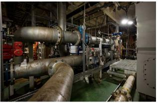
Forward ballast water treatment system installation (Photo courtesy A&P Australia)
