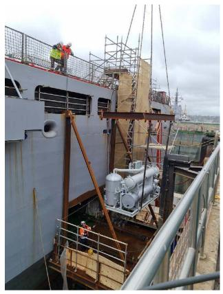
Hanging platform welded to ship's side for aft chiller installation (Photo courtesy A&P Australia)
