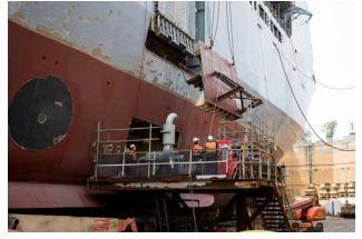
FFG platform in use on HMAS *Choules* (Photo courtesy A&P Australia)
